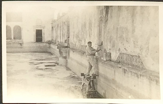
Repair of wall and tiles by lake -- about 1938
