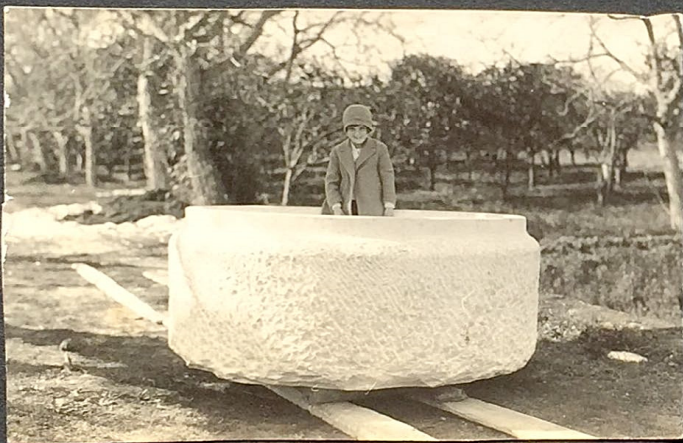
Circular bathtub before it was hoisted into tower. Probably 1937.
