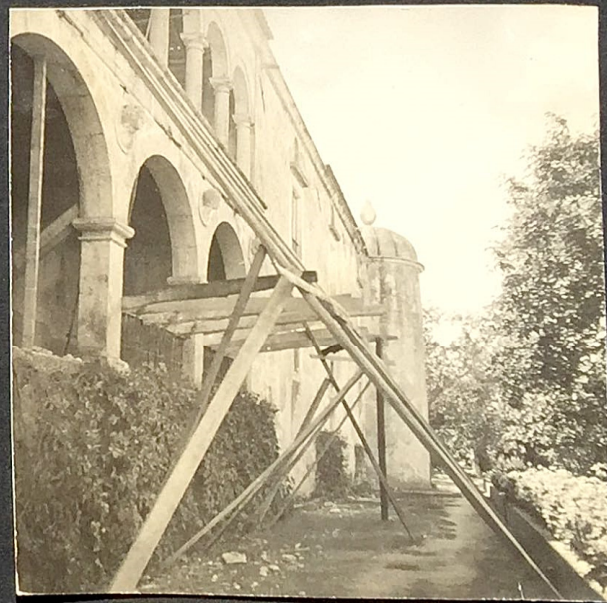
Restoration of north side of house -- 1937
