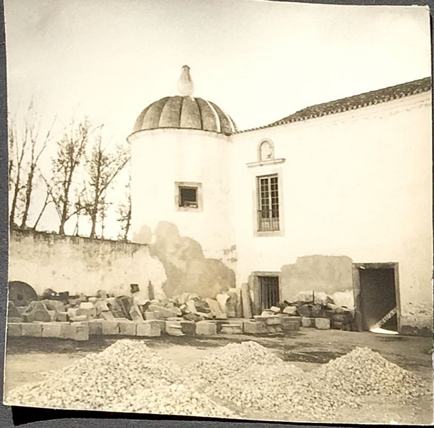
Photos taken during restoration work 1937
