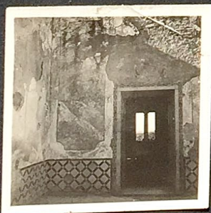
Music room looking toward the living room. Taken in 1937 before restoration. Note the original wall mouldings to the left of the door but now covered over with plaster. Similar moulding is on wall where the large box bush is next to the topiary box garden.
