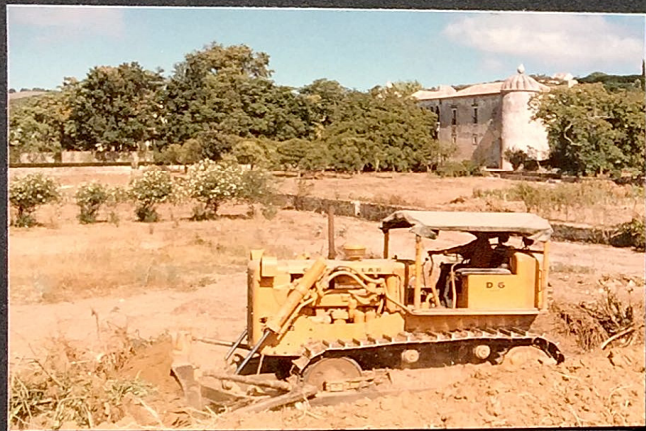
Vineyard construction -- August 1974
