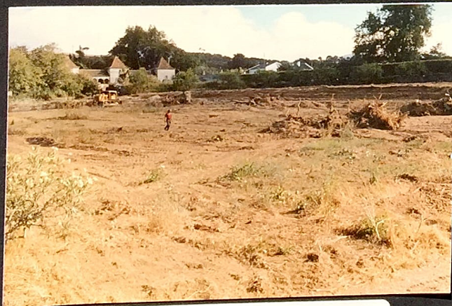
Vineyard construction -- August 1974
