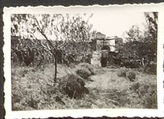
Tower along wall before restoration. 1937 or 1938.
