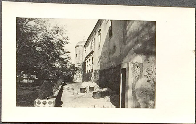
Arranging tiles on north side -- probably late 1930's
