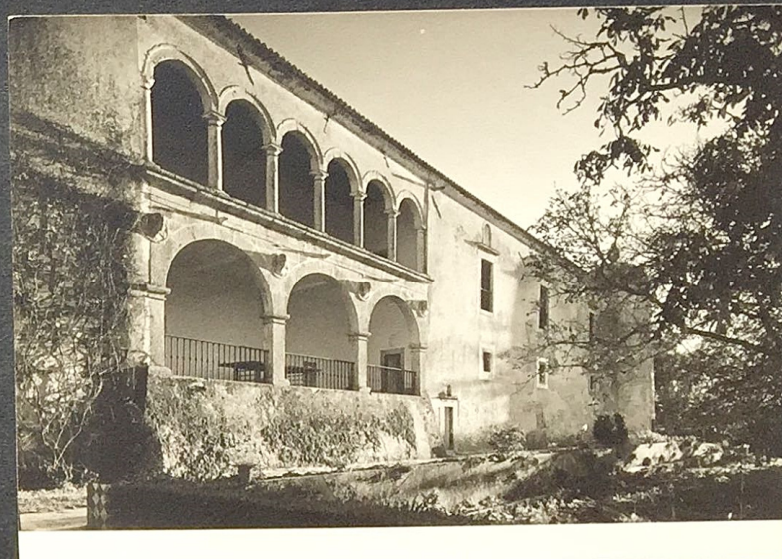
Completed restoration of north side. probably early 1940's
