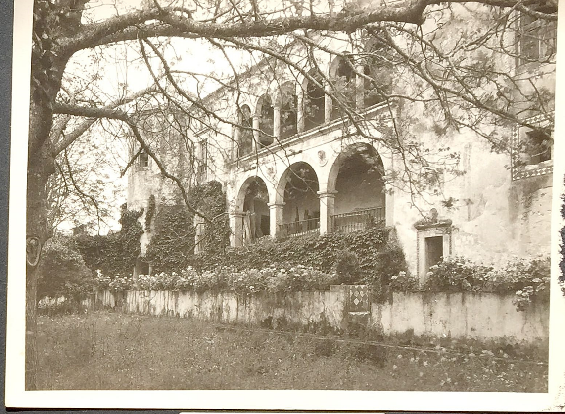
North loggias before restoration -- 1937
