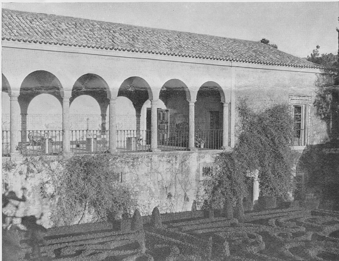
5.—THE WEST LOGGIA. Its seven pillars are made of multi-coloured local marble
